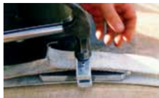
2. Close clamp plates with a hammer protecting the tank with a block of wood.
