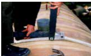
7. Continue rotational tightening until strap is snugged down.
