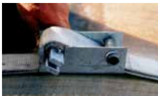
4. Insert gal. Bolt Spacer and rotate clamp to take up slack strap. Place guides x (2) on strap.
