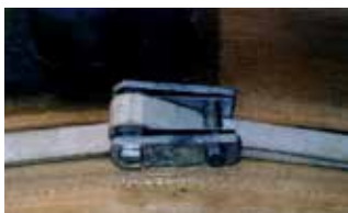
10. Bolt fully tightened and clamp complete.
