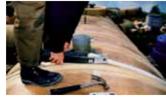
6. After each crank hold position with one spanner and reposition one at a time.
