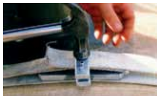
2. Close clamp plates with a hammer protecting the tank with a block of wood.
