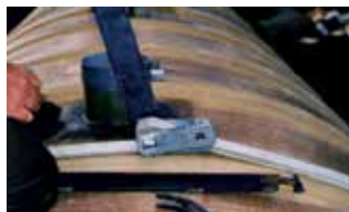
8. Assemble side holding plates over clamp ends, use spanner on the outside to locate & align assy
