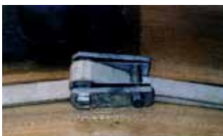
10. Bolt fully tightened and clamp complete.
